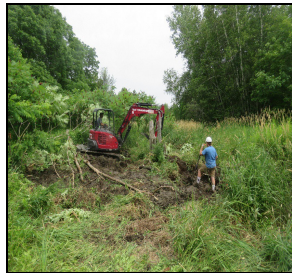
Nathan and Nikolis clearing vegetation with an excavator. Photo: Laurie DiCesare
