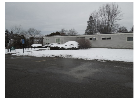
Blundell House Photo: Michael Sabourin
